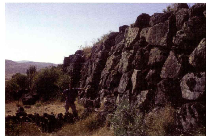
Fig. 5: Close-up view of main wall at Dumanlı Kale, showing batter and saw-tooth steps in alignment.
