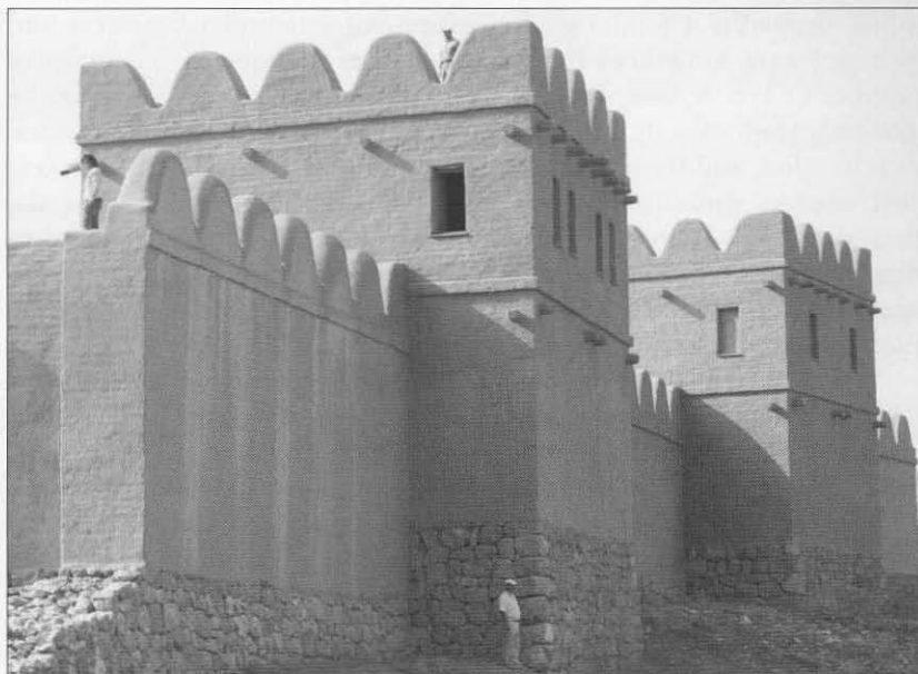
Hattusa fortifications, as recently reconstructed. Note the mudbrick construction on a stone foundation. (Courtesy Deutsches Archäologische Institut – Istanbul)
