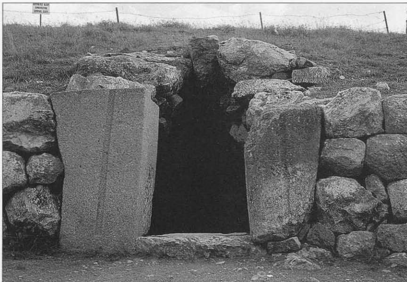
Postern gate. Postern tunnels were a typical feature of Bronze Age fortifications. They provided the defenders of a city with access to and exit from it during a siege, either for gathering provisions, or for making surprise attacks upon the enemy. The external gate to the postern in the south wall of Hattusa is shown here.
