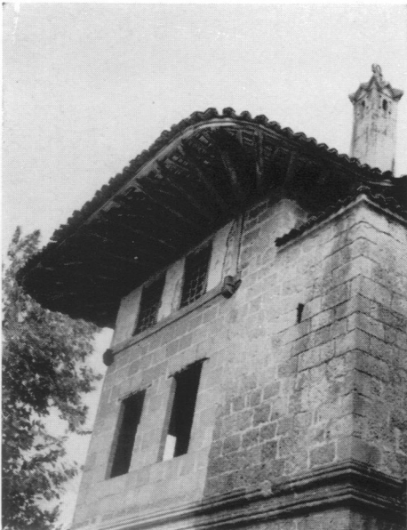
(b) Oblique view showing the overhanging eaves and a modern repair of masonry in the north-west angle.
