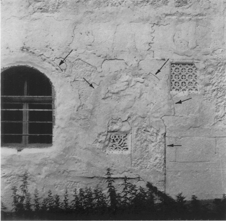
(a) St. Philip, part of west wall showing blocked opening.
