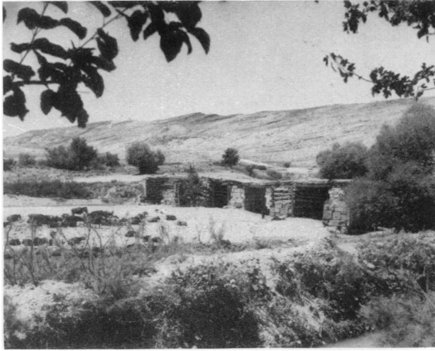
1. Bridge at Sykeon.
